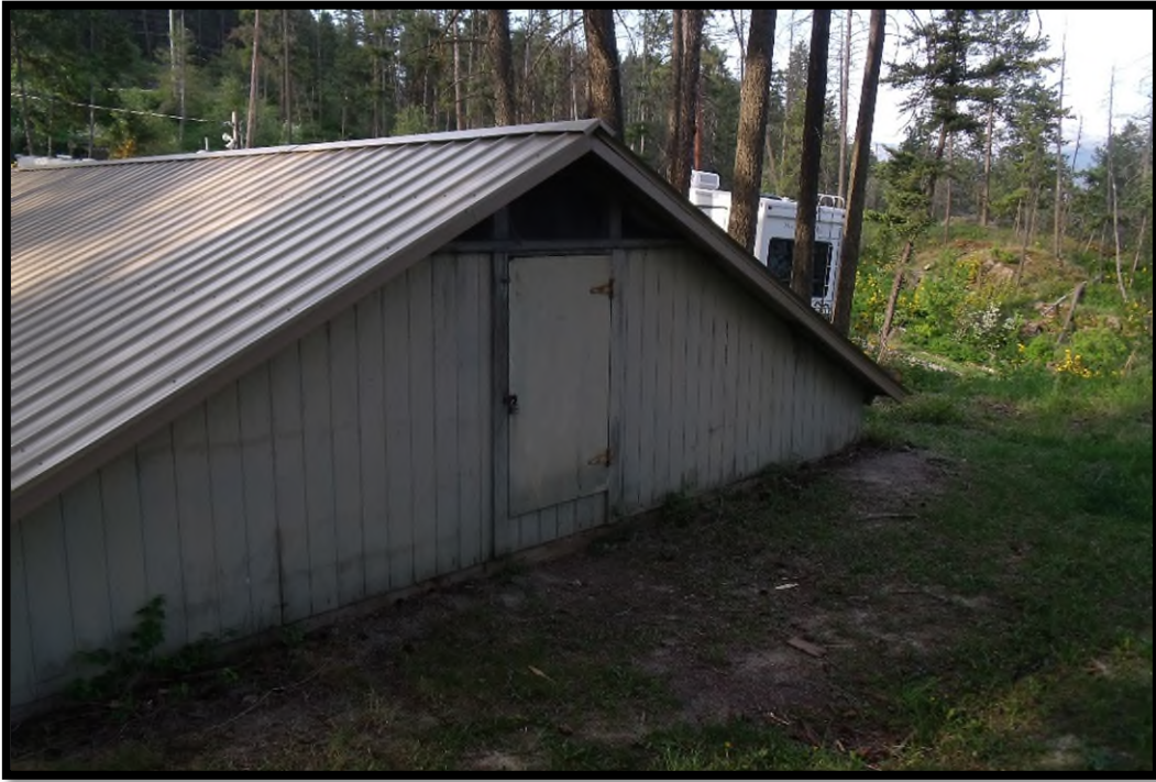
Figure 1 Delcliff Covered Reservoir
