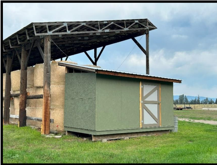
The finishing and painting of the storage shed at the park.
