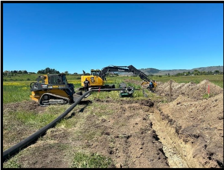
New irrigation installation
