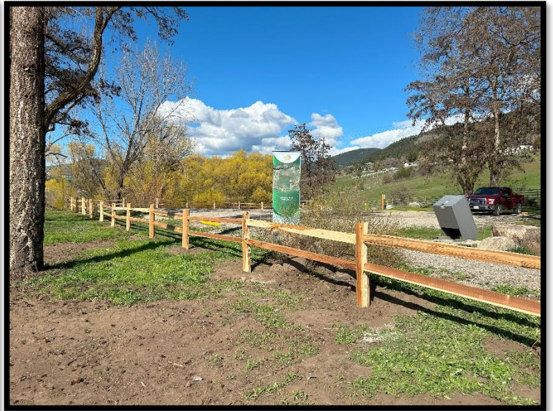
Parking lot post and rail fence construction & installation
